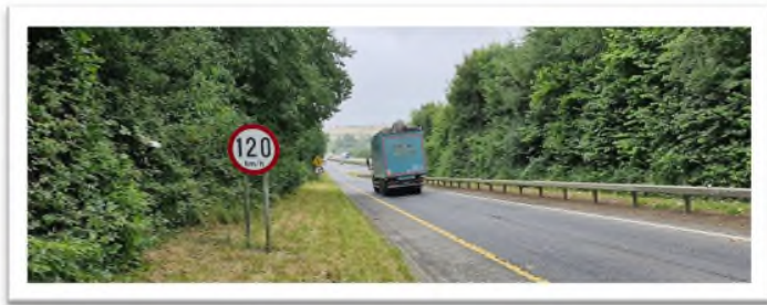
120km/hr section of M1 slip
