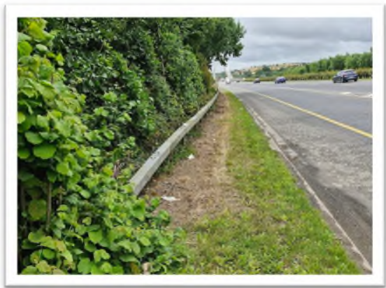
Approach OBB to parapet Railing over Old Slane Road.
